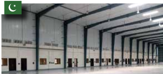
Air Force hangar Pakistan | HANGAR
